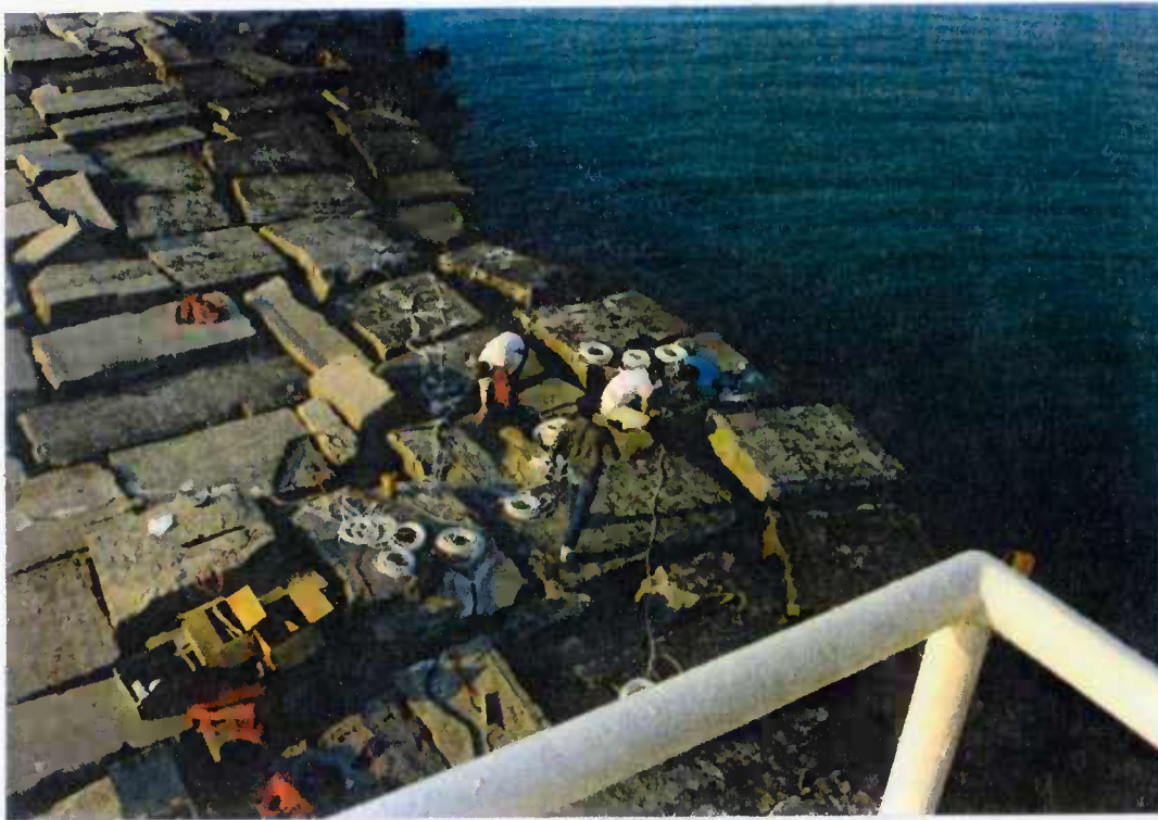
Fig. 2.3. Layout of instrumentation Cable network
