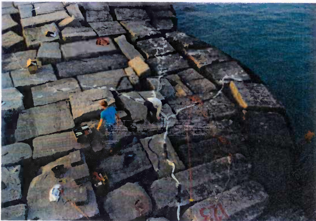
Fig. 2.6 Final stages of the installation operation
