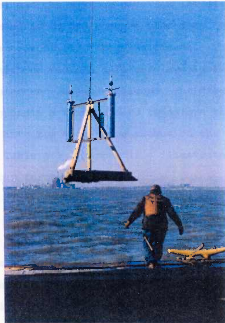
Fig. 2.9 Wave gauge being installed at site by the Corps of Engineers personnel
