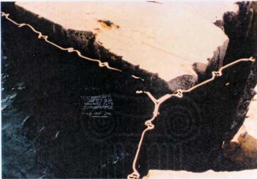
Fig. 1.6. Plan view of a cell indicating split piles at a Y - Intersection
