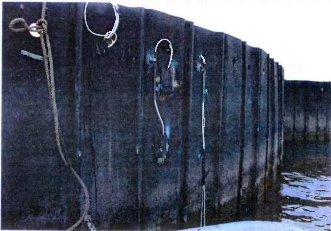
Fig. A.4. Angle barriers welded to strain gauges 2 and 4
