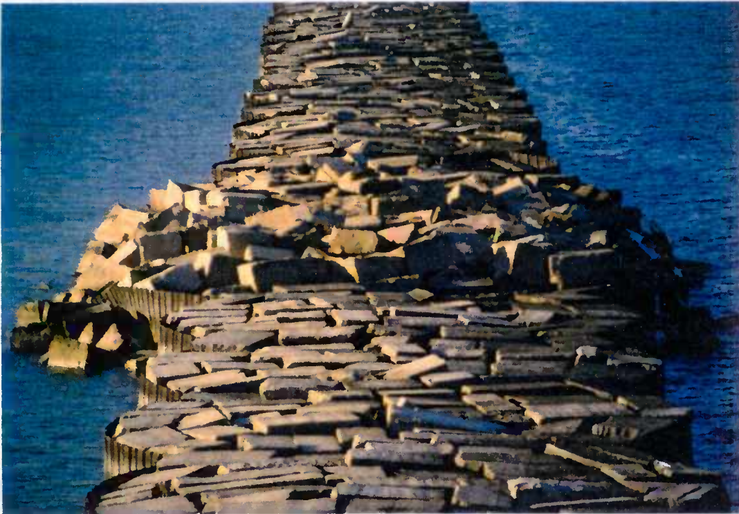
Fig. 1.8. Photograph of rubble mound created at cells 115, 116 and 117
