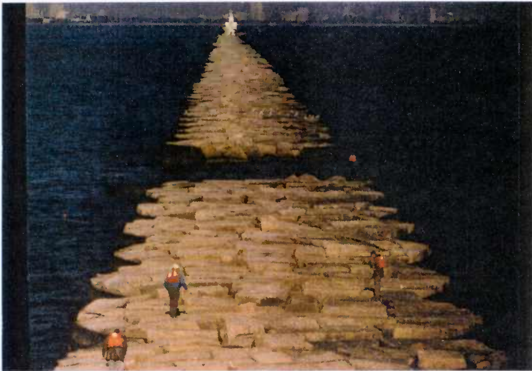
Fig. 1.5. Photograph of the failed cells during a reconnaissance survey
