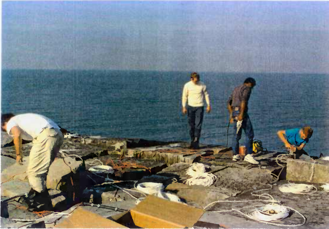
Fig. 2.5 Fixing of cables to capstones
